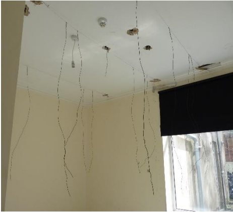
Holes made in ceilings to locate rafters for lamp fixings
