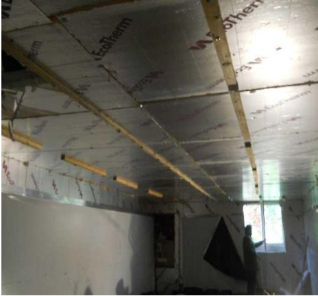
Room lined with insulation material
